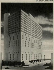
An operations center for Manufacturers Hanover Trust Company, New York (left), designed by Carson, Lundin & Shaw, is a 22story structure with a brick exterior to relate it to nearby brick landmarks. The architects said that the Stockholm City Hall was the reference point for the design of the building. The building, scheduled for occupancy in 1969, will contain 800,000 square feet.
