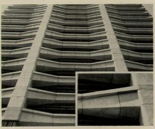
White cement and white quartz sand combine to create a bold sculpture which dramatically defines the individual "work areas" of the office building. Tinted glare-reducing glass contrasts sharply with the white concrete frame. The frame segments were cast in Tedlar-coated steel molds resulting in dimensional accuracy and uniformity of color and texture. The precast concrete exterior surface is permanent and will require little or no maintenance.
