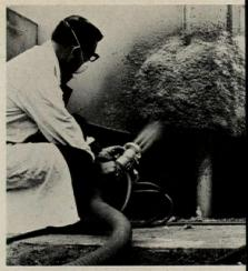
INSULATION / Two spray mixes (one for 2200 F and one good to 1350 F) go on at 600 lb/hr with no nozzle clogging and low rebound loss. Application technique permits rapid insulation of industria equipment. Both mixes provide a laminate construction which permits varying of wall thicknesses. The Babcock & Wilcox Company, Augusta, Georgia.
