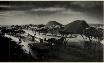
Second prize design by Whittlesey, Conklin & Rossant, has only one structure above grade, the roof of the indoor riding ring. Described by Mr. Conklin as "mountain-like landscape forms," the 40-foot-high roof structure has compression rings at the top engaging radial steel columns. Surfaces between the steel radials are formed of concrete with slate. At top of the conical shapes are skylights.
