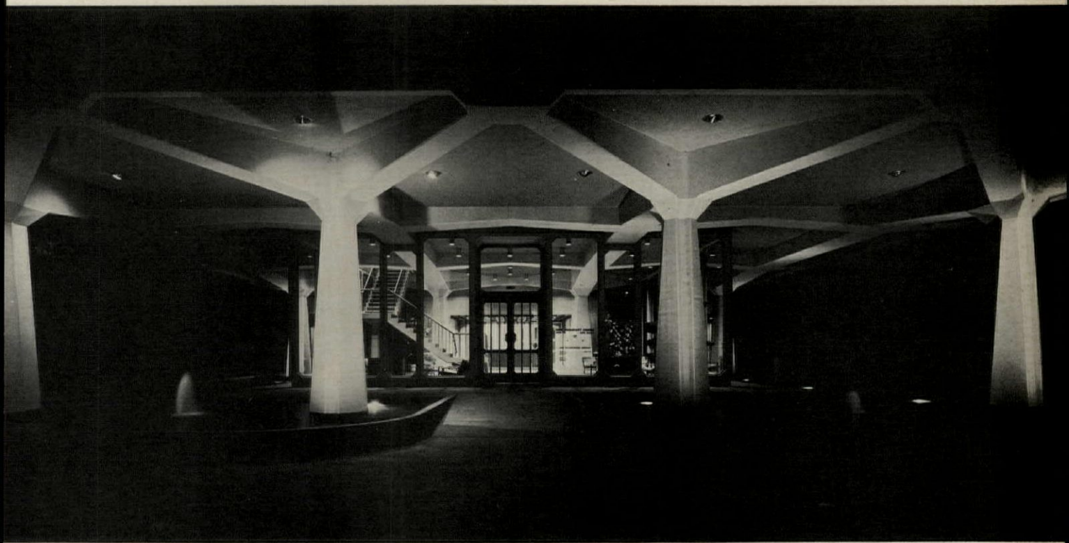
The concrete sunshades which cut the air-conditioning load, and the pools on either side of the entrance in which the columns stand along the front of the building are distinctive features of the design. The building won a design award from the Seattle Chapter of the A.I.A.
