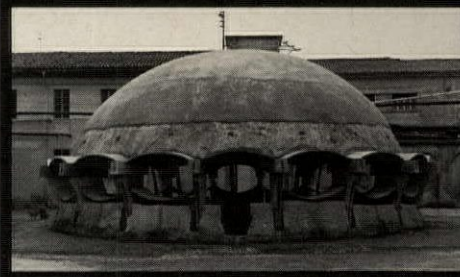
Balloon-formed concrete dome was erected at Columbia University last month by first laying reinforcement (spring-like coils plus bars) over an inflatable membrane which was tied to a perimeter ring. After concrete was placed, a different membrane was laid on top to help maintain evenness of the concrete as the balloon form was inflated. Photos left and right are of structure in Italy, illustrating openings cut out of the dome after construction.
