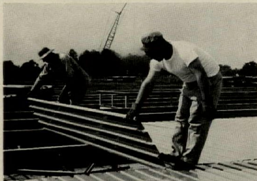
ROOF DECK —strong, lightweight steel decks in a selection of five patterns and six gages for every roof construction need.
