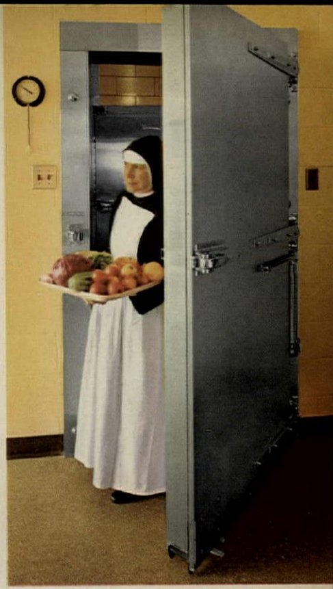
Cooler door with automatic closer.
