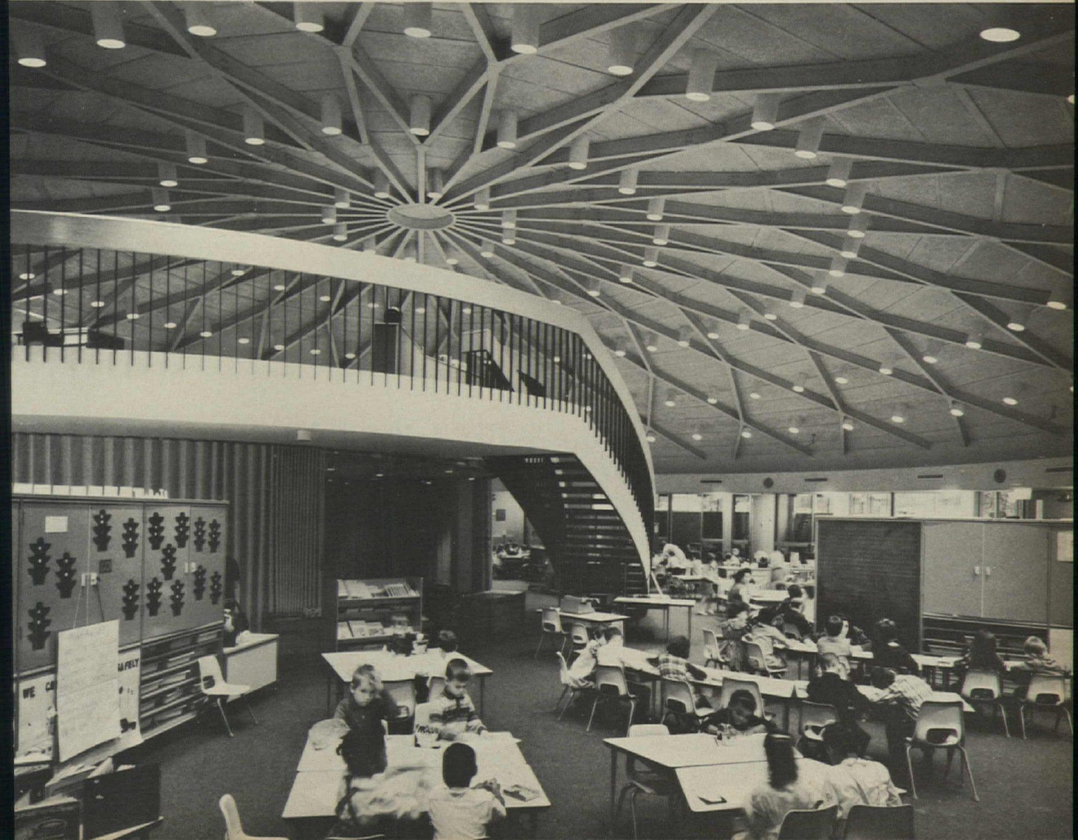
The big open space under the lamella dome in this satellite K-2 school can be sub-divided by informal dividers for class groups. All furniture is also movable for flexibility. Lead curtains are provided around the central "learning arena" for soundproofing when the area is used for noisy activities. Sound absorbing materials are also used on floors, ceiling and dividers. One-way windows let observers watch class instruction.
