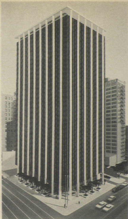
Illinois Bell Telephone Company Architect: Holabird & Root
