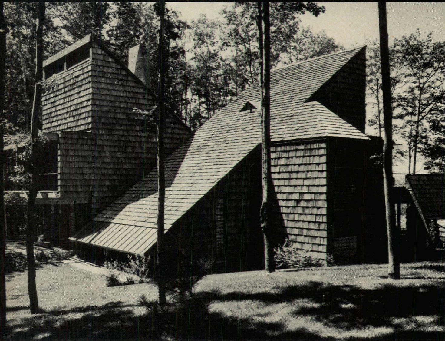
Residence, St. Bruno, Quebec | Architects: D'Astous and Pothier | Certi-Split Handsplit-Resawn Shakes, 24" x 1/2" to 3/4" with 10" to the weather on sidewalls and roof.
