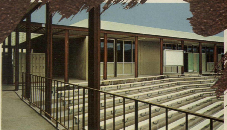
Dos Pueblos High School photographed 10 months after erection. Architect: Cooke, Frost, Greer & Schmandt, Santa Barbara, California. Structural Engineer: Stanley H. Mendes, Santa Barbara, California. General Contractor: James I. Barnes Construction Company, Santa Monica, California. Structural Steel Fabrication & Erection: Griffin Fabricators, Inc., subsidiary of Griffin Steel and Supply Co., Inc., Bakersfield, California.
