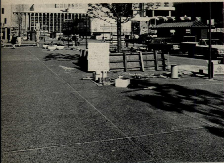
The terrazzo-surfaced mall is divided into snow melting zones, with high wattage mat installations located near stores and at corners for pedestrian
