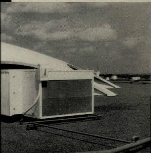
Design Concepts, John H. Glenn Junior High School, San Angelo, Texas: Plan view, above, shows how modern concepts of team teaching, flexible scheduling and individualized instruction find architectural accommodation. Roof mounted air conditioning equipment, with multizone distribution, permitted designers to eliminate "walls" of space and time. Thus, the building anticipates innovative teaching concepts of the future, as well as housing those of today. ARCHITECTS: Donald R. Goss Associates. ENGINEERS: Cowan, Love & Jackson, Inc.
