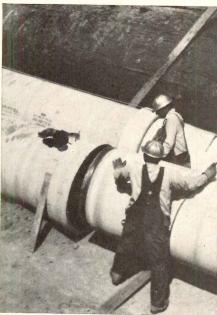
Century City chose J-M TRANSITE\* asbestos-cement pipe for both chilled water supply and return lines. TRANSITE resists corrosion inside and out...features J-M Ring-Tite® joints (coupling with rubber rings) for water-tight seals, elimination of expansion joints, quick and easy assembly. Some insulation value. Lower installed cost, but higher operating costs than with but higher operating costs than with insulated J-M Temp-Tite.
