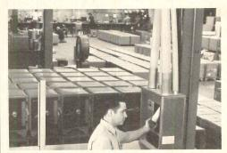
AIR CHUTE / Cutler Air Chute is said to move materials up to 25 lbs at speeds up to 35 miles per hour economically and safely within or between hospitals, office buildings, retail stores and similar buildings. The air envelope is generated by a low power blower system which conserves the heated or cooled air it draws into the tubes. There is no need for an air make-up system nor is additional load placed on the heating and air conditioning system. Cutler-Federal, Inc., Rochester, N.Y.
