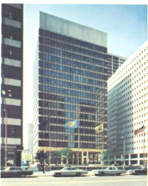
21-story IBM Building, Philadelphia (15 glass-enclosed office floors). Offset service core (not shown) serves as the backbone and steel framing serves as the rib cage to provide unusual openness and flexibility of space. Corrugated steel underfloors contain built-in channels for telephone and electrical wires. Architect: Vincent G. Kling, FAIA.
