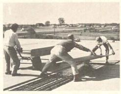
ROOF INSULATION / Fiberglas roof insulation comes in a new large size that is said to sharply reduce installation time and cost. The four-ft by eight-ft insulation, with a thickness of 1 5/16-in., does not sacrifice thermal efficiency, but rather has the same "C" values as two-ft by four-ft insulation boards. • Owens-Corning Fiberglas Corporation, Toledo, Ohio.
