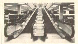
MOVING WALK / Movator, a two-way moving walk system, is used in Montreal's new Steinberg's-Miracle Mart. The treadway, at a 12-degree incline, is of grooved rubber bonded to a three-foot-wide spring steel belt. It is 78 ft long and travels at 120 ft per minute. Balustrades are of 1/2 -in. hardened and tempered safety glass.
