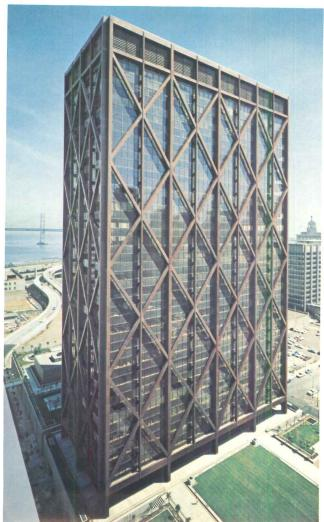
24-story Alcoa Building, San Francisco. Steel diagonal bracing, together with vertical hangers and only twelve exterior columns, form a sophisticated system for resisting seismic forces. Floors, column-free except for the service core, are suspended within the clad steel frame. Architect: Skidmore, Owings and Merrill.
