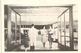
AUTOMATED ENTRANCEWAYS / Two features of a new line of air doors are the recirculation of air in a closed system and a patented sensing system that automatically changes the direction and velocity of the downward flow of air to offset change in outside wind velocity or interior air pressure. The Stanley Works, New Britain, Conn.
