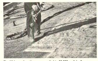
The 1" layer of urethane was applied to 98,000 sq ft by 3-man crew. Foam was later sealant-coated for added durability.
