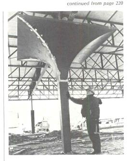
STEEL COLUMN SHELLS / Flaring column shells at the Inland Steel Company's new Employees' Credit Union Building, Chicago, are designed by the architects, Richard E. Glass & Associates. Shells carry live wind loads up to 35 pounds per sq ft and enclose three-inch XXH steel pipe columns which carry the entire dead load of the roof structure. Inland Steel Company, Chicago.
