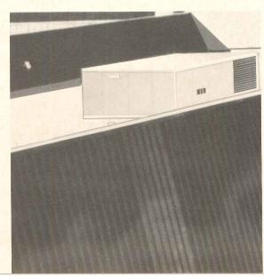
◀ In Freeway Office Park, buildings have handsome copper mansard roofs which provide all-weather protection for walkways. Their slight rise above normal roof line is sufficient to conceal the Lennox DMS units that deliver 350 tons of cooling and 6,000,000 Btuh heating for the
