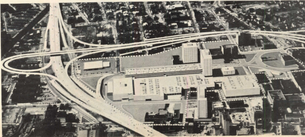
Lafayette Plaza Bridgeport, Connecticut Architect: Lathrop Douglass
