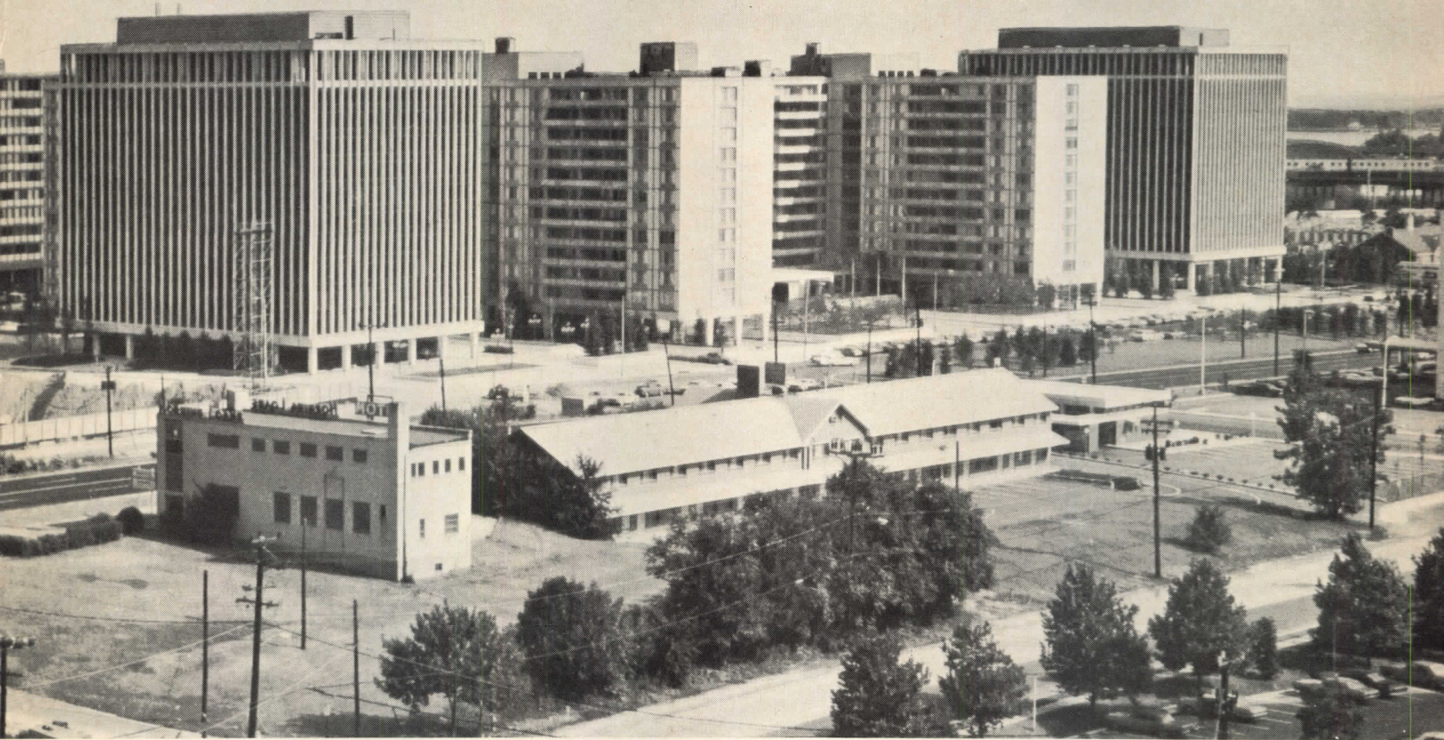
Ceco Steelform Service for 790,000 sq ft of monolithic concrete joist construction 12,700 tons of Ceco-fabricated Reinforcing Steel 480,000 sq ft of Cecocolor Anodized Aluminum Windows and Curtainwalls
