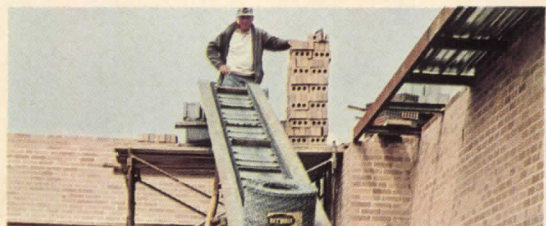
Keywall Multibond comes in rolls that are easy to hand carry, roll, convey, or wheel. One roll reinforces 200 ft.
