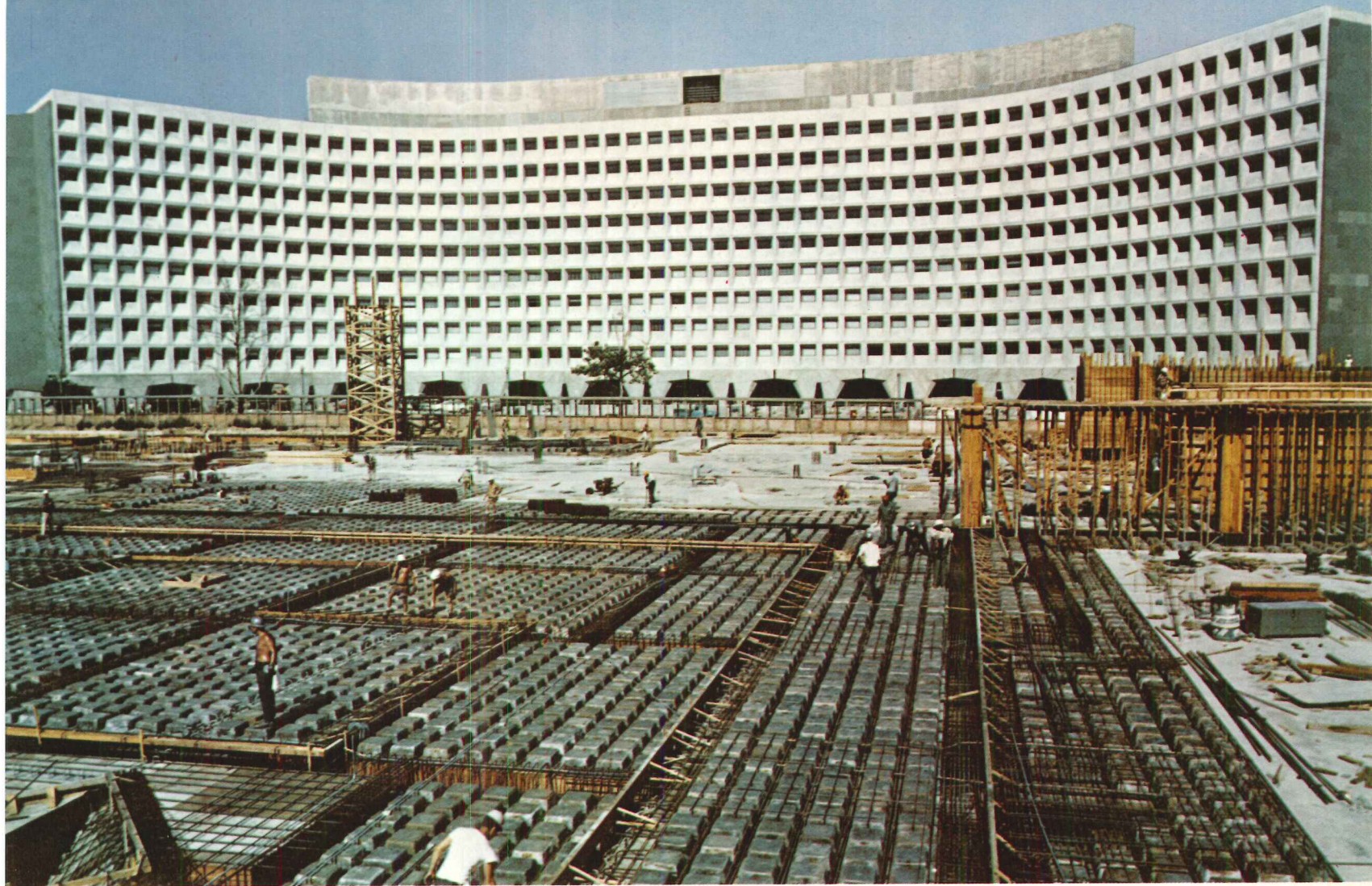
Foreground: Construction of Nassif Office Building, Washington, D.C. 2,000,000 sq ft of Ceco Steeldome Services David Nassif Associates, owner / Edward Durell Stone, architect Universal Engineering Corp., engineers John A. Volpe Construction Co., Inc., contractors Kirk Lindsey, Inc., concrete contractors (Background—National headquarters building of HUD also utilized Ceco's experience in forming reinforced concrete joist construction for central core.)
