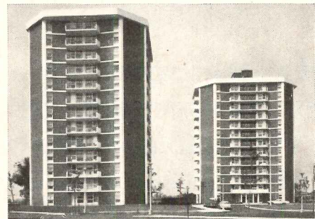
Stephen J. Collins Elderly Housing "Twin Towers" Architect: Caolo & Bieniek Associates Engineer: Greenleaf Associates
