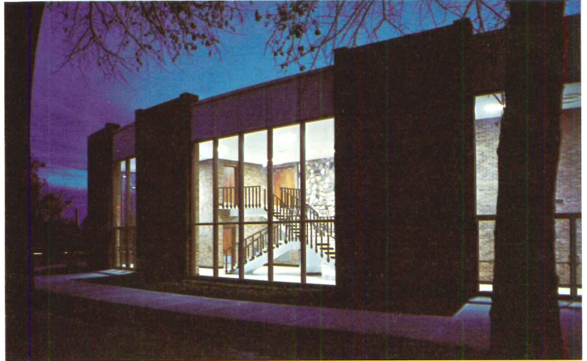
Clafin University, Fine Arts Building, Orangeburg, South Carolina Architect: Godwin & Beckett
