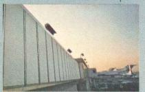
by combining the best features of precast concrete and nickel stainless steel. Architect and client can be confident that the wall will be free of corrosion streaks for the life of the building.
