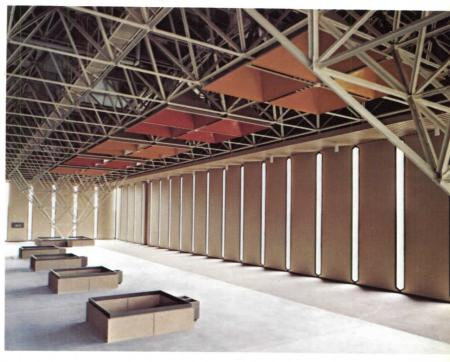
H. H. Robertson Company textured and shaped the panels to add warmth and shadow effects. Weathering steel plate was used to frame each window. Mel Elward Company assembled and erected the wall panels.
