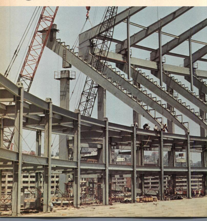
strength structural bolts were used to fasten intermediate beams on upper levels.
