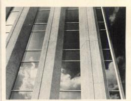
COATED GLASS / The 2300 West Loop Building in Houston was recently completed using Vari-Tran/Chrome coated glass for all vision and spandrel areas. The glass was chosen because of its "environmental control characteristics of reducing heating and cooling loads and for visual comfort." The sky and surroundings are reflected in the glass. Libbey-Owens-Ford Company, Toledo.
