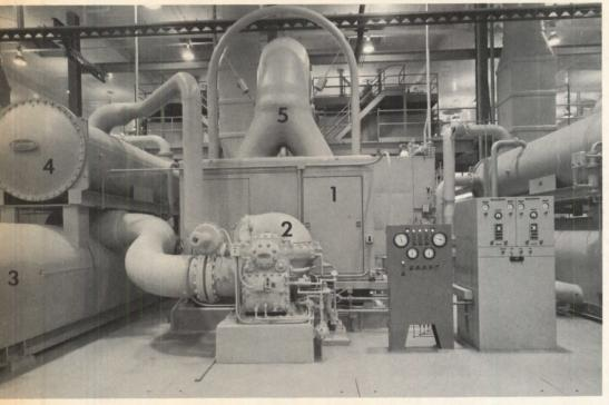
Numbers on the photos and on the drawing, right, identify principal pieces of equipment producing motive power and refrigeration: 1. dual gas turbine drive, 2. refrigerant compressor, 3. water chiller, 4. refrigerant condenser, 5. gas turbine exhaust, 6. heat-recovery boiler. The top photo shows the doors open on the soundattenuating cabinet of the gas turbine unit. Heat recovery boiler is behind the turbine unit in the photo directly above
