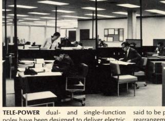
poles have been designed to deliver electric power and communications wiring to outlets where there are no walls, where floor outlets are impractical and where the methods and materials used must harmonize with modern office decor. The system is
