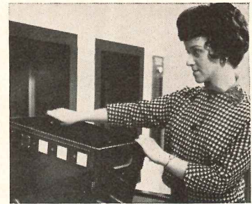
At proper floor, the box is automatically shunted off vertical conveyor. "Magnetic memory" control system has no moving parts, levers, or between-station wiring... nothing to wear out.
