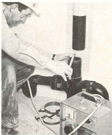
Polypropylene fittings and pipe for chemical wastes quickly joined with electrical fusion process.
