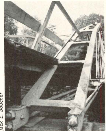
Cast iron bridge, circa 1860, near Albany, N.Y.
