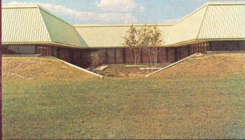
1. RCA Graphic Systems Division Plant, Dayton, N.J.
