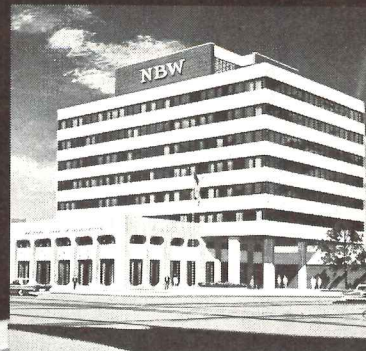
Laszlo Papp and Associates, architects; R. C. Daly, construction consultant; Alexander-Jennings Construction Co., general contractor; Consolidated Stone Setters, setting contractor.
