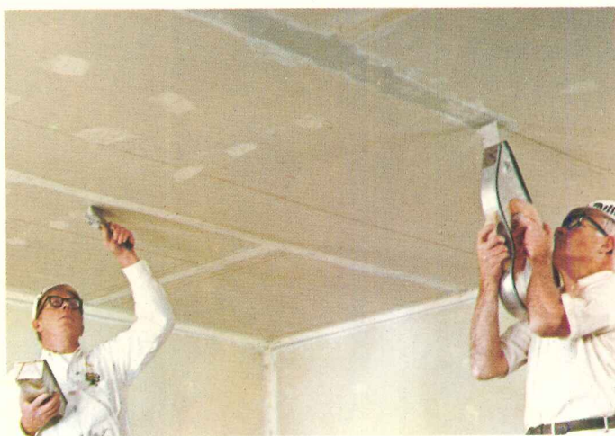
Panelectric panels are factory-wired single-layer \frac{5}{8} " Fire-Shield Gypsum Wallboard, and can be applied, papered, painted or textured like any other gypsum board ceiling.
