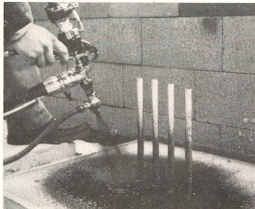
Seamless membrane goes up to and on pipes and conduits.
