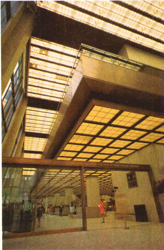
The bronze lobby ceiling lights, which can be seen from the exterior, complement the overall building design.
