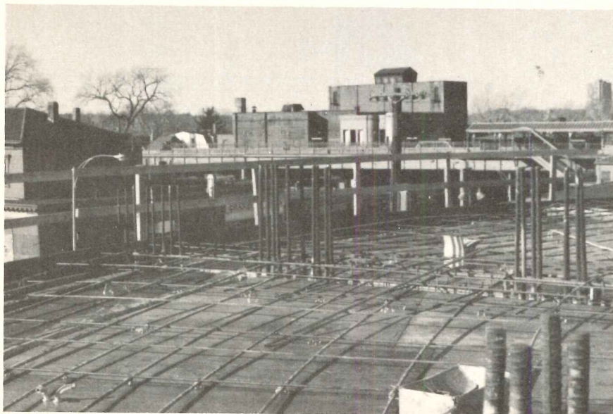
Grid of curved prestressing beams and of three of the supporting columns can also be seen. Just over half of the slabs have been post-tensioned and de-centered in the photo, right.
