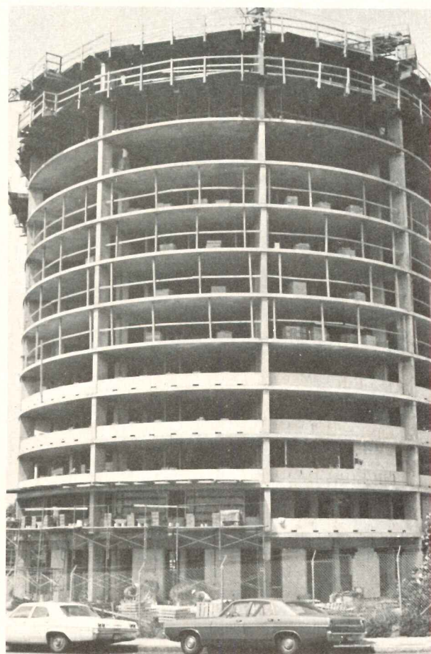
Grid of curved prestressing beams and of three of the supporting columns can also be seen. Just over half of the slabs have been post-tensioned and de-centered in the photo, right.
