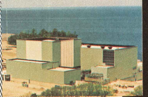
1. Ginna Nuclear Station, Rochester Gas & Electric Corp.
