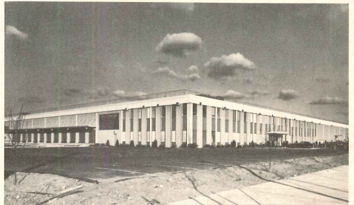
Times Square Stores General Offices and Warehouse, Flatlands Urban Industrial Park, Brooklyn, New York. Architects and Engineers: Engineers Incorporated of Newark; Dr. Jacob Feld, New York, Consulting Engineer.
