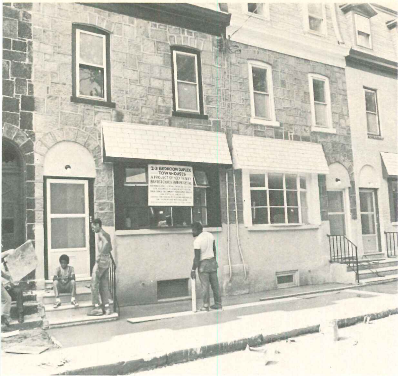
Philadelphia Gus Baxter, Executive Director of the Architects Workshop, is shown above left, outside the renovated main office in central Philadelphia. The Wayneview Apartments, left, is a forty-unit building being rehabilitated under FHA 236. Under the supervision of Workshop architects E. J. Messersmith, W. Gray Smith and W. E. Kramer, half of the units have been completed. Two of the five Holy Trinity Baptist Church duplexes renovated by the Workshop and architect John Fatula under FHA 235 are shown above.
