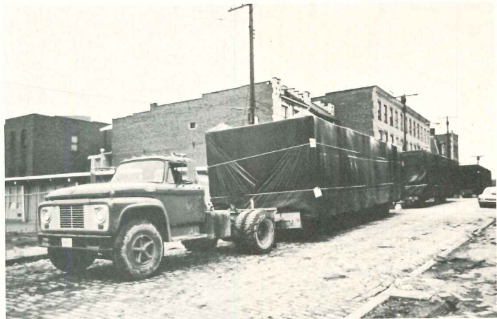
Nine modules are stacked longitudinally to form six apartments at each end of a building. Each three-bedroom unit has an outside module and shares an inside wet module (one is about to be lifted into place, bottom) with its neighbor. The space between the two stacks becomes a stairway shared by both. Two two-bedroom apartments of masonry construction form the base for the modules, making a total of 14 units per building.
