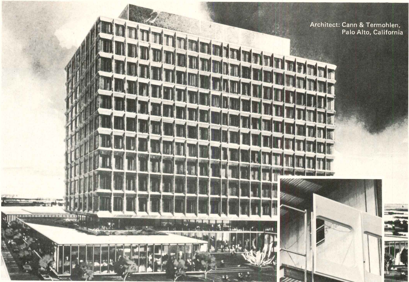
Fiber glass panels clipped to steel frame on third floor of IED Building.
