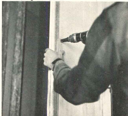
3. Attaching core to T-spline.
