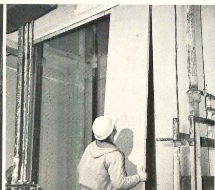
2. Installing core panel.
