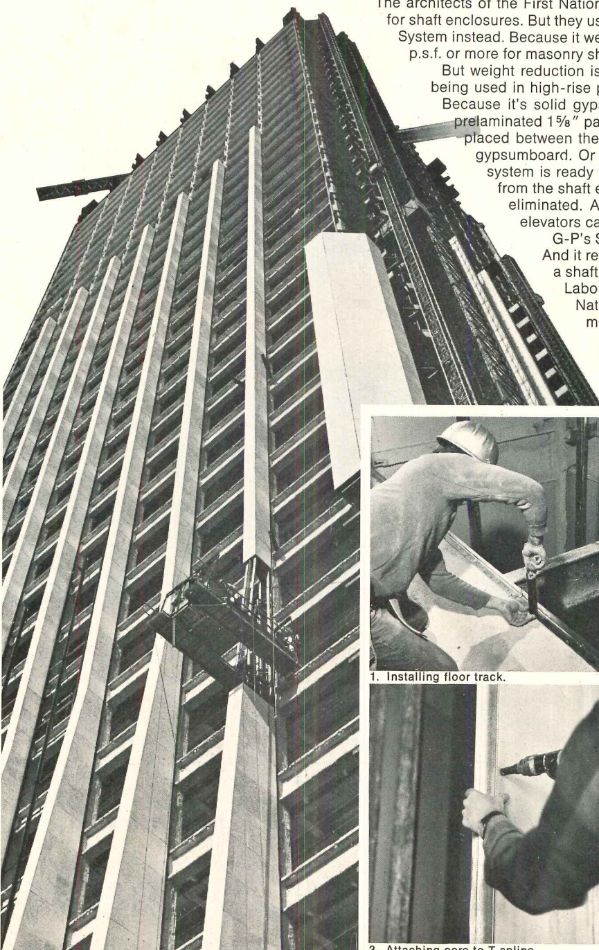
3. Attaching core to T-spline.
