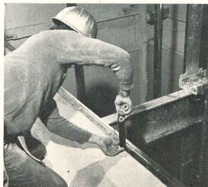
1. Installing floor track.
