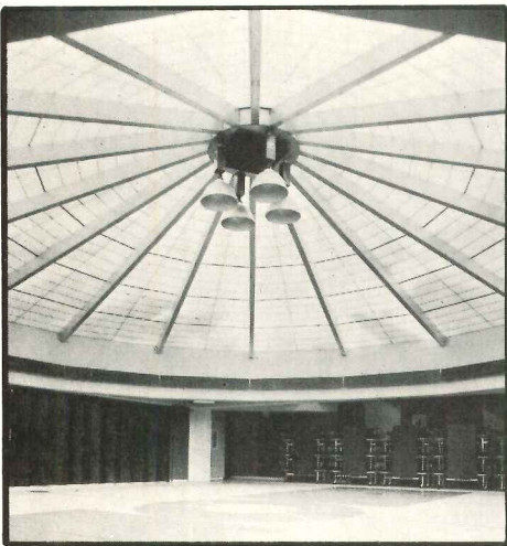
2¾" translucent Kalwall Roof System at Summit School in South Dakota.
