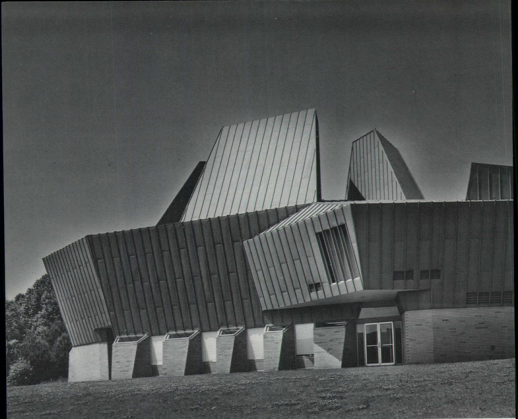
Congregation Beth El, New London, Conn.; Architect: Paul Rudolph, FAIA, New York, N.Y.; Roofer: H. R. Hillery Company, Groton, Conn.
