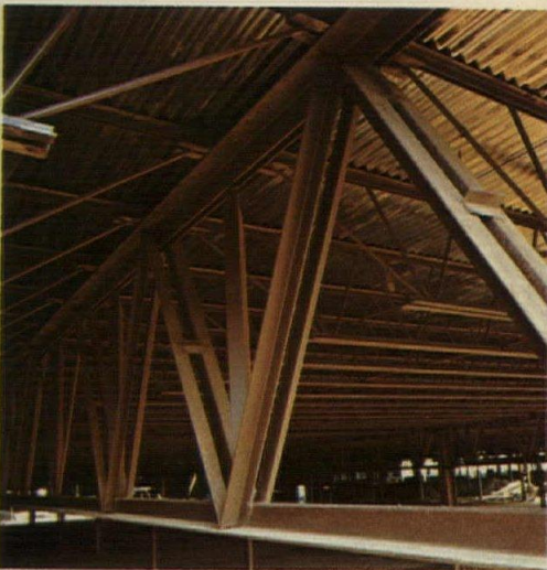
Joist girders have a modified Warren truss configuration using hot rolled double angle sections for top and bottom chords and single and double angle sections for web members. What that means is a high strength to weight ratio.
