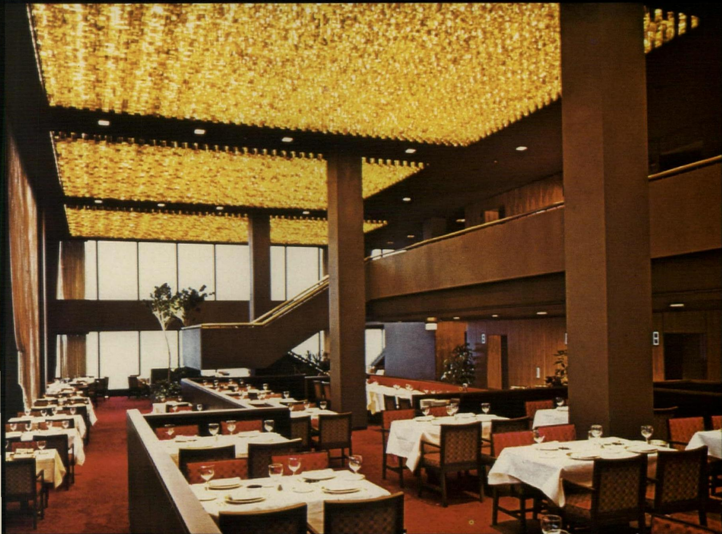
Leaf-Lite Ceiling in Muntz Metal John Hancock Building, Chicago.
