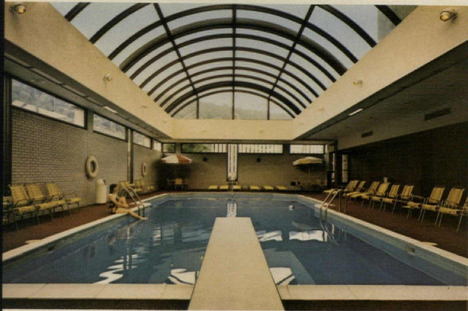
Major clear span area in the first floor is over the pool. This enclosure measures 45 by 74 ft. The next major span is over the largest of the four meeting rooms, which measures 36 by 64 ft. This room can be evenly divided by a movable partition.
