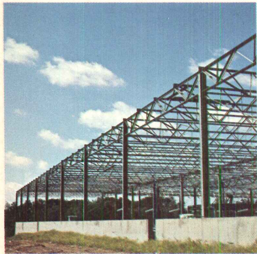
Joist girders have a simple span design. Which explains why ponding calculations are easier. And why design time is shortened.
