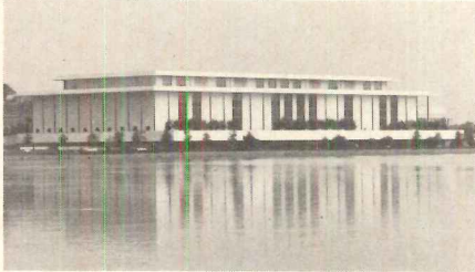
John F. Kennedy Center for the Performing Arts, Washington, D. C. Architect: Edward Durrell Stone, New York, N. Y. Acoustical consultant: Dr. Cyril M. Harris, New York, N. Y. General contractor: John McShain, Inc., Arlington, Va.
