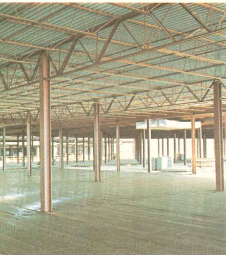
Joist girders need fewer foundations and columns. Which means less work for you and larger savings for your clients.
