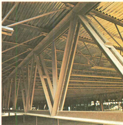
Joist girders have a modified Warren truss configuration using hot rolled double angle sections for top and bottom chords and single and double angle sections for web members. What that means is a high strength to weight ratio.
