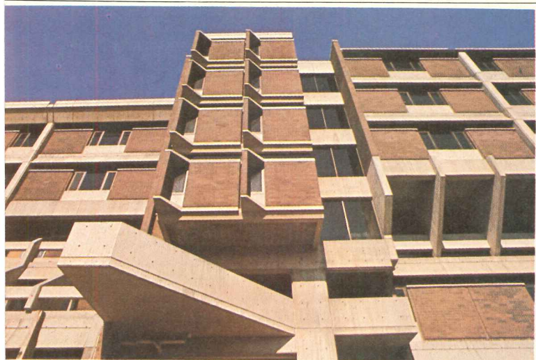
The physical education plant (above) has a full-size gym on the top floor with a competition-sized pool below. Fenestration changes with room size function and orientation as the photos on this page indicate. The triangulated windows increase the apparent size of small faculty offices. The peace symbol (bottom), cast in concrete, places these buildings firmly in their time.
