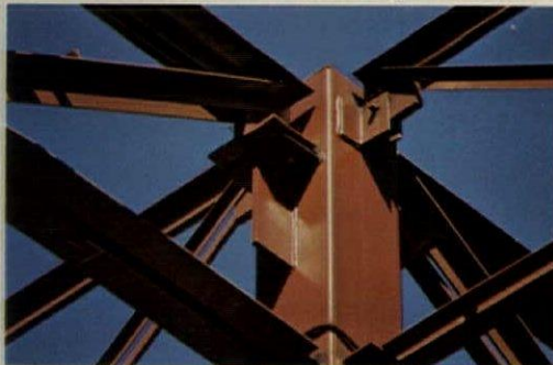
The standardization of column connection also speeds up construction. And requires fewer connecting bolts.
