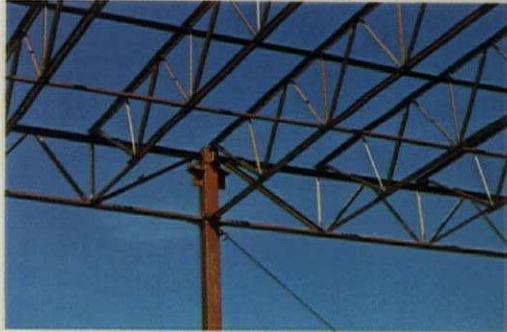
Vulcraft's steel joists and joist girders allow a standard five-foot module between connecting points.
