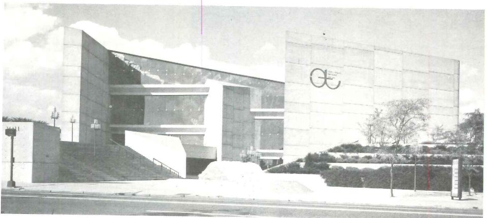
EDWIN J. THOMAS PERFORMING ARTS HALL , Akron, Ohio. Jury Comments: "Extremely competent in the planning and use of the site in a congested urban area... achieves human scale." Owner: University of Akron, Akron, Ohio. Architects: Caudill Rowlett Scott, Houston, New York, Los Angeles, Dalton, Van Dijk, Johnson & Partners, Cleveland, Ohio. Structural Engineers: R. M. Gensert and Associates, Cleveland, Ohio. General Contractor: Mosser Construction, Inc., Fremont, Ohio.
