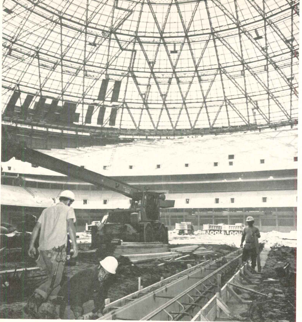
Movable stands on each side of the field, weighing almost 1000 tons each, are supported by pipe frames that sit atop caterpillar-type roller assemblies in tracks recessed below the floor.
