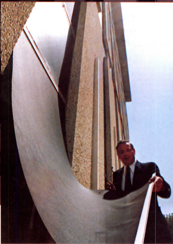
Phil Iatesta, Chief Engineer of Bethesda (Md.) Air Rights Building, shows how easily solar screen unlocks for window cleaning. He expects payback through energy savings in less than two years.
