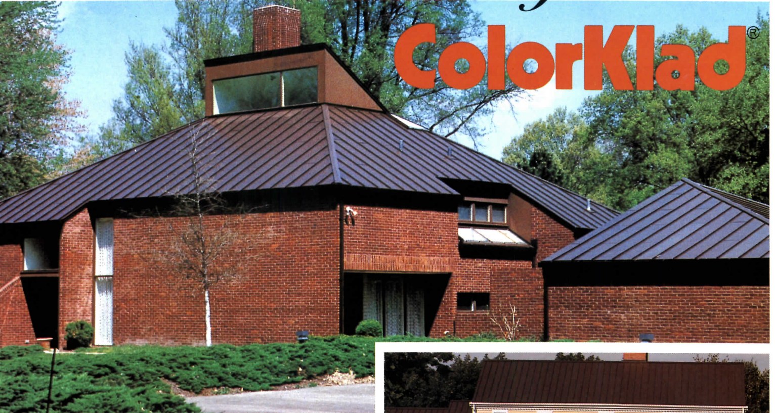
Sheet metal contractor — Zero Breese Co., Cincinnati, Ohio.
