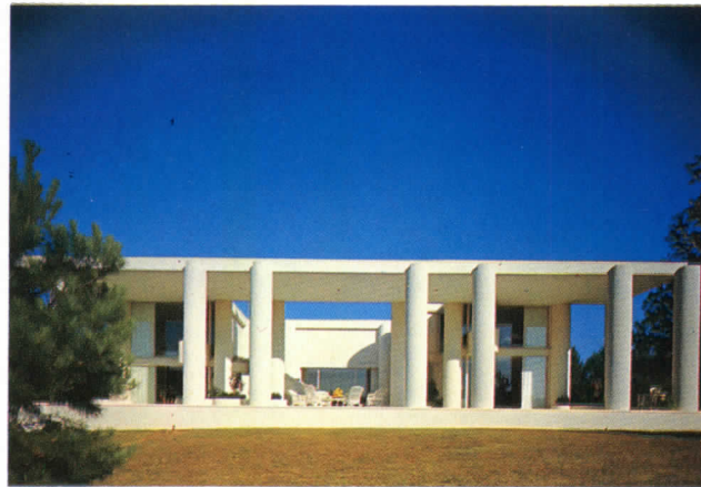
Far left: Government Service Center, Boston, Massachusetts, by Paul Rudolph (1962-1968). Left: Wallace House, Athens, Alabama by Paul Rudolph (1961).
