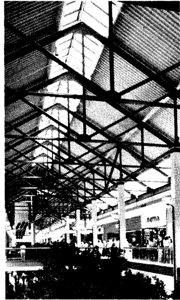
elements as trees, brick paving, park benches, a town clock, and decorative columnar lighting reinforce the image of a main street. Exposed structural steel used in the fabrication of the skylighted roof evokes the steel trusses and corrugated metal decks of Baltimore's old waterfront buildings. The AISC jury cited the roofing system in particular as the element that "animates an otherwise conventional way of treating a shopping center."
