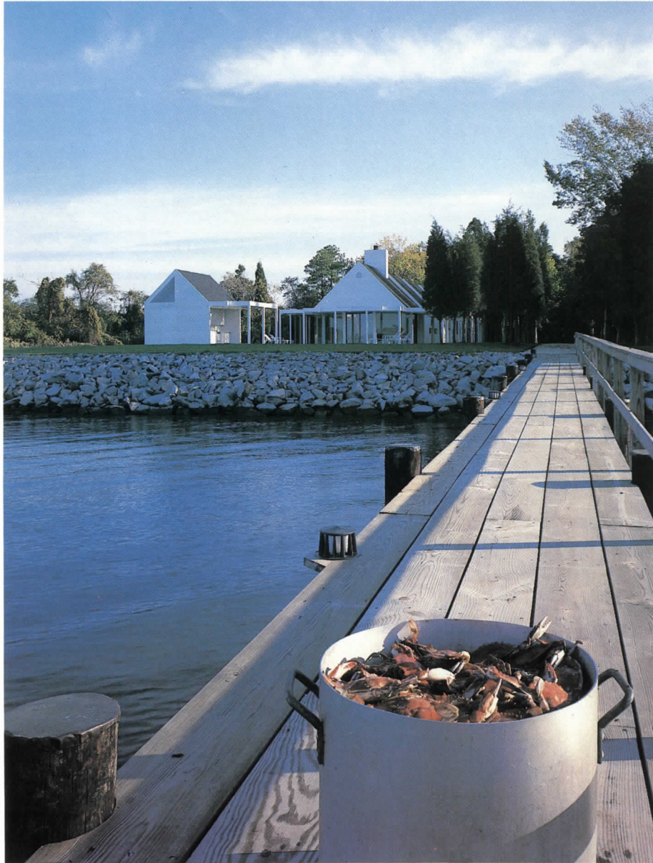
Modest, and quite “Eastern Shore” in its appearance, the real scope of the house—and even the large parking lot—are artfully screened by trees. What looks as if it has always been there, but was indeed planned, is seen above and the drawing top left.
