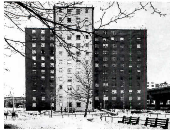
Thacher Homes in Albany before (small photo left) and after (large photo) rehabilitation by architects Crozier Philippi Associates. Members of the project team included J. Gregory Crozier, Thomas C. Glynn, Stephen R. Griffing, Charles G. Siconolfi, and Gerald W. Spillane.
