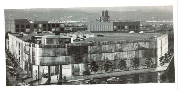
Tanner & Van Dine Architects is testing Nippon Electric Glass Co. details for elimination of vertical mullions to enhance seismic safety in the DataMart building under construction in San Francisco. About 18,000 clear glass blocks will be used in the curtain walls.
