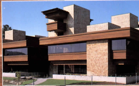
Architect: Lawrence Simons & Associates Project: Waterfall Towers Office Park Photo: Karl H. Riek
