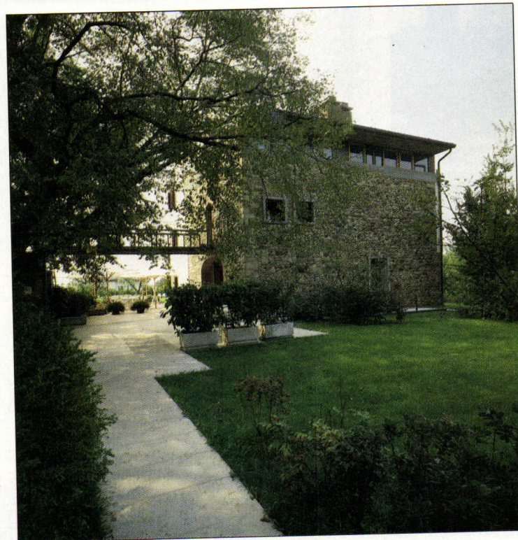
One of the most striking materials introduced at the farmhouse during restoration was a locally-quarried stone, pietra di prun . The stone was used outside to pave a walkway and a patio that wraps around the building on three sides, (opposite page and above). Inside pietra di prun was also used as a flooring material and for the sensitively detailed stairs (overleaf).
