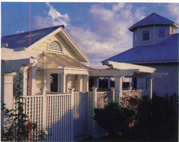
A tentlike gazebo and solar-heated sauna flanked by pergolas rise above low-lying undergrowth to form Rosewalk's civic heart (preceding pages). In order to focus a forced perspective of upper Rosewalk from an entry gate along county route 30A, the architects positioned a pair of tower houses on opposite sides of a north-south garden axis that narrows as one advances toward the center of the complex.
