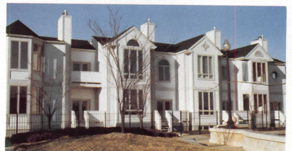
Wilkins-Riedmann & Associates, Inc., Frank J. Riedmann, Architect
