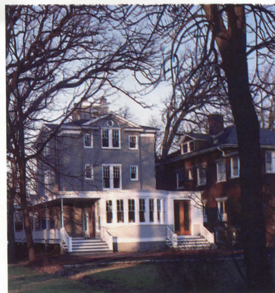
Street and side views of the Hansen House (top and facing page) reveal a villa-like monumentality that relates to the ample scale of its neighbors. By contrast, the rear elevation (above), with its asymmetrical juxtaposition of porch and door openings, is meant to address a different context—the frequently haphazard rear alterations and additions on nearly all the adjoining properties.
