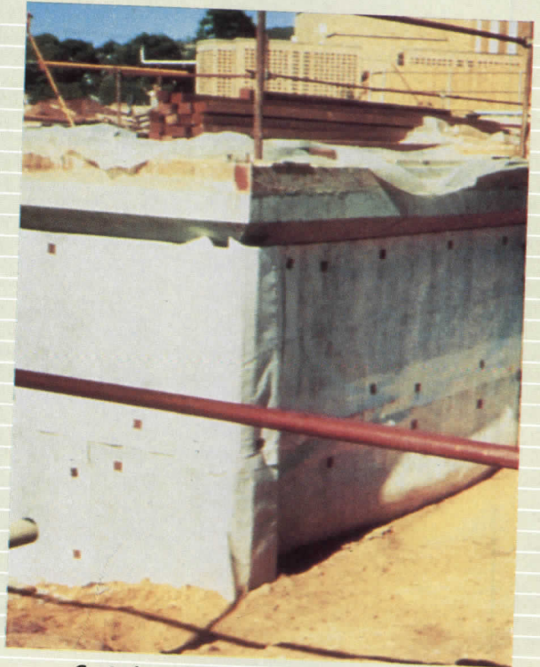
Contech STRIPDRAIN 75 drains more water than a 14'-thick sand or 17"-thick gravel drain.
