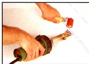
Hand-welding a field seam in a confined area.
