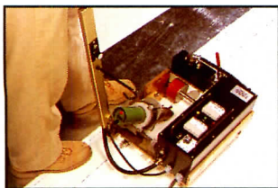
Self-propelled, hot-air welding machine fuses HyChoice seam.
