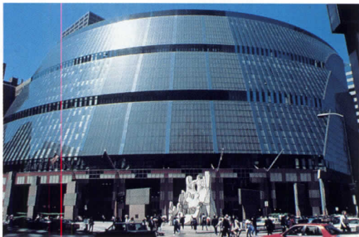
State of Illinois Center
