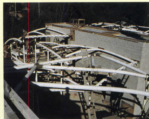
The south terrace (top drawing) and view north from the entrance (bottom drawing) are shown above. Steel elements, which Holl calls “noddles in space,” form a frame of doubly curved metal roofs, shown under construction (above).
