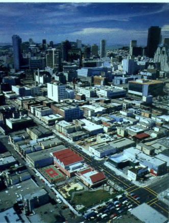
The Sixth and Folsom Community Center (bottom in aerial photo) is a green oasis in the tightly packed urban web of South of Market, "an area of complexity, tradition, and transition" in the architects' words. The center's multi-function program was developed through a series of participatory meetings during which the community evaluated alternative uses and site plans. In a sand-filled play area local children produced a path that passes ceramic sculptures designed by San Francisco artist Martha Heavenston (opposite).
