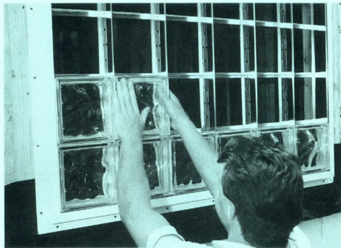
316 Glass-block installation grid. The IBP pre-framed aluminum grid eliminates the need for traditional mortar laying up of all thin-series (3 1/8-in. thick) glass block patterns, making for a much quicker and more uniform installation of walls, skylights, and floors. The biggest standard-size grid is 96- by 144-ins., which can be mul-tioned together to create larger panels. Perforations in the grid insure good contact of the silicone sealant. Acme Brick Co. Product News continued on page 133
