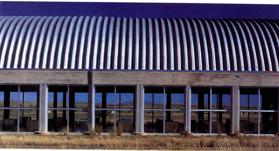
Judd added corrugated iron barrel-vaulted roofs and aluminum-framed square windows to former artillery sheds.
