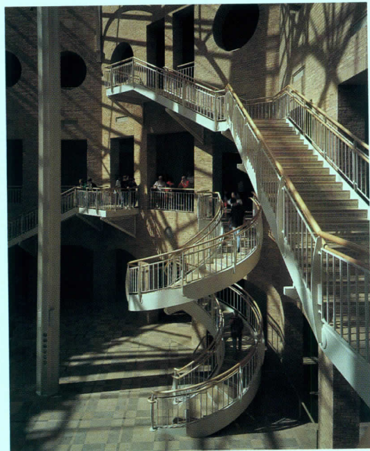
Steel columns (top) sprout like trees in the octagonal "Great Hall" and exfoliate into trusses that support a glass roof and pattern the interior with shadow. Steel stairs (above) climb the wall. Floor plans (right) show how the Great Hall serves as the major organizing element for the three-story interior. Permanent exhibits, the cafeteria, and access to the IMAX theater are at entry level. Special exhibits are below, while workshops and childrens' area are above.
