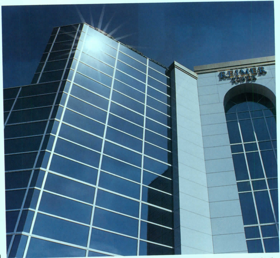
The Reimer Tower in Burlington, Ontario features VISIONWALL curtain wall without any form of perimeter heating.
