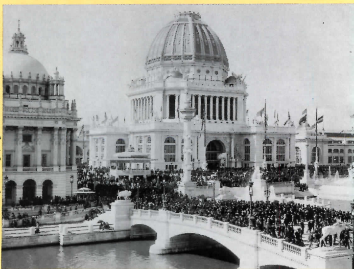
Grand Plaza in front of Administration Building.
