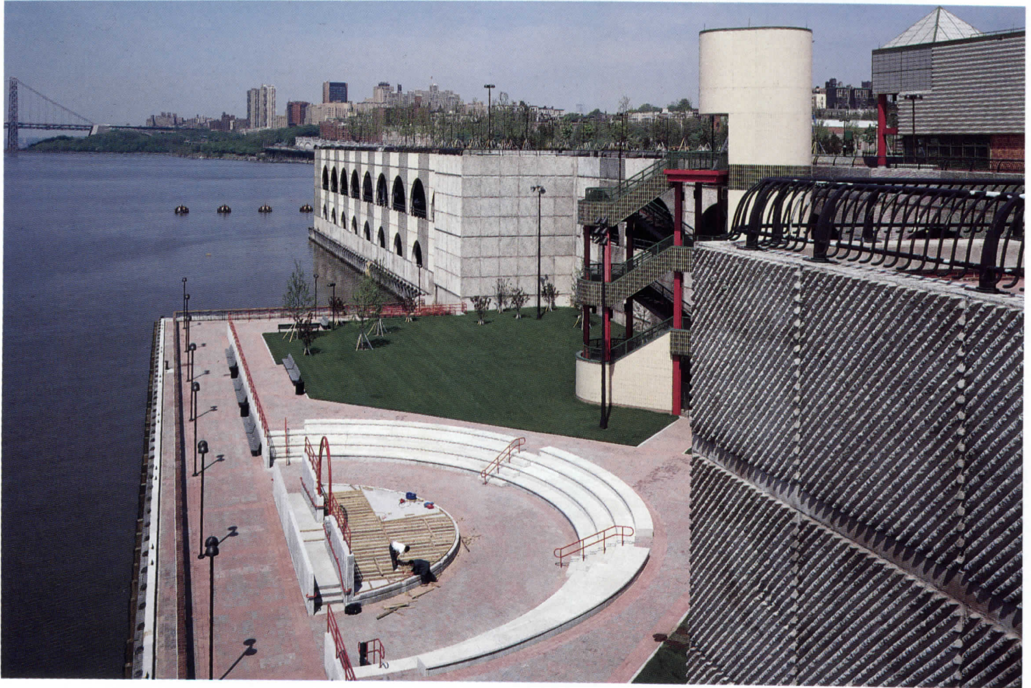
Most of Riverbank State Park is 58 feet above the river. An exception is the Amphitheater and promenade (above) located only a few feet above the waterline of the Hudson. It is isolated to keep noisy events from disturbing neighbors to the east. This level is accessible via the stair/elevator tower in the center of the photo.
