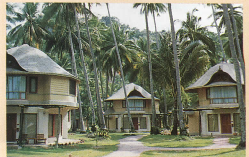
At the Dusit Rayavadee resort in Krabi Province, Four Aces designed buildings that echo traditional Thai architecture and fit sensitively with the jungle (below).
