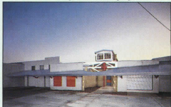
1. 8522 National Boulevard Complex (exterior); phase I, 1986-1988 [RECORD April 1988, pages 90-97].
