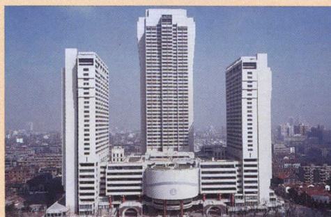
Two by ECADI: Bank of China Headquarters, Shanghai, with Callison (top); Shanghai Centre, with Portman (above).
