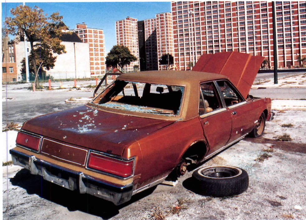
The Corbusian idea of towers in a park has been subverted into towers in a parking lot, with abandoned cars dotting the landscape.
