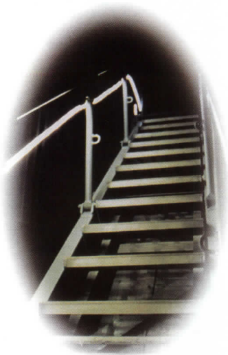
U.S. Naval Ship Accommodation ladder
