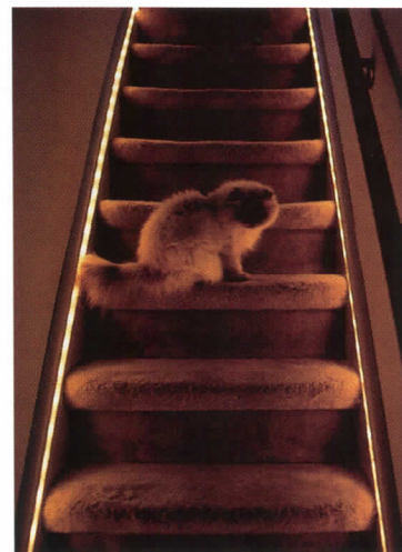
Low-voltage light strips on the stair risers are activated by a concealed motion sensor. The cat is an optional component.
