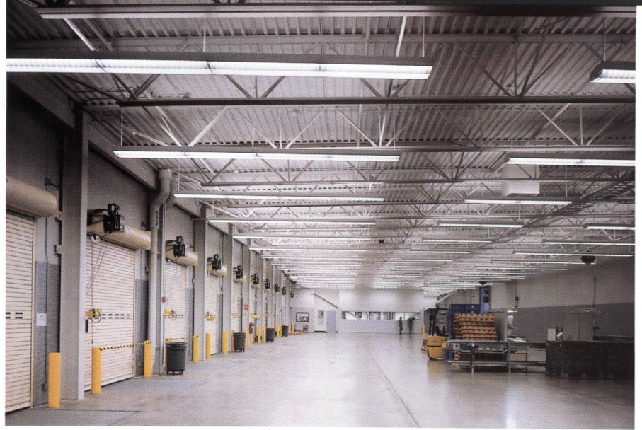
In the warehouse, left, forklift operators moving materials on pallets need to be able to read shelf labels quickly. In the shipping area, above, light from the luminaires reflects off white-painted ceiling, trusses, and walls to produce very uniform illuminances.
