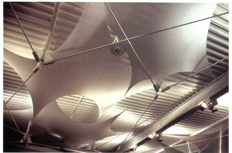
The shape of the fabric reflector/shade was fine-tuned using a model (left). A detail of the finished shade (right) shows the soft, indirect light produced by the system.
