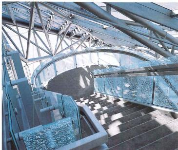
Glass panels, which have a layer of fractured glass sandwiched between two unbroken layers, reinforce the
