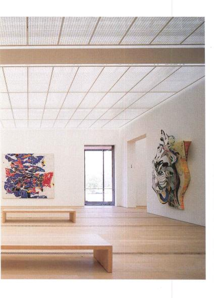
The visual permeability of the metal-mesh ceiling makes for a livelier experience than that offered by the windowless "white cube" spaces the Beyeler's galleries resemble.
