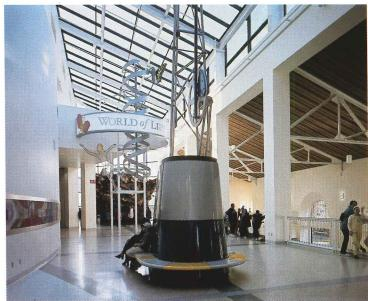
Exhibit spaces are grouped around the central atrium. Steel trusses, remnants of the 1913 structure, are
