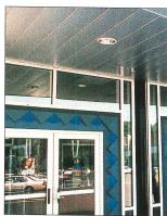
This revolutionary ceiling system offers nominal 12" (300mm) wide panels in lengths up to 19' 8" (6m) creating a clean, sophisticated, monolithic ceiling plane. Long spans are available with a soft beveled edge or a reveal edge. The system provides both acoustics and aesthetics with easily installed panels. Available in 8 finishes and 2 perforation patterns. For further information call 800-366-4327.
