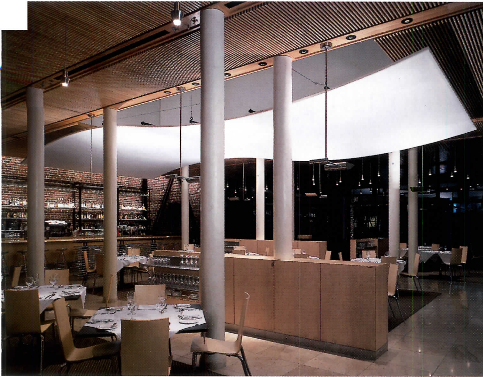
Stainless-steel pendants uplift a wave-shaped metal frame covered with scrim fabric. Twenty-watt
