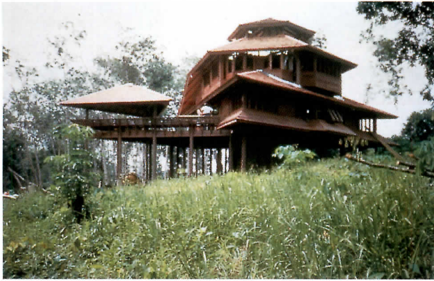
Salinger Residence, Selangor, Malaysia Architect: Jimmy C.S. Lim
