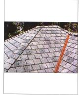
An oversized 18" x 36" fiber glass asphalt shingle designed to withstand hurricane force winds. Features a dramatic eight-inch exposure; deep oneinch shadow lines; seven colors; and a 40-year limited warranty, including 10-year warranty coverage against winds up to 110 miles per hour, the highest of any fiber glass asphalt shingle on the market today. UL certified to meet ASTM D3462 performance standards; Miami-Dade approved; algae resistant.
