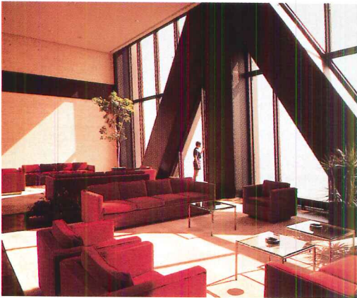
The megascale exposed steel structure with diagonal reinforcing members has a powerful presence on the exterior (above and right), and at key points on the interior (below).
