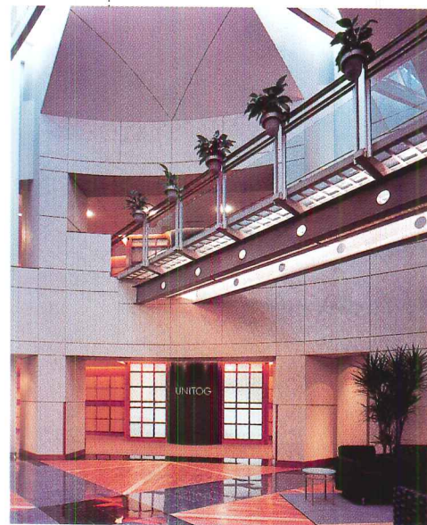
Skylights trace the top chords of the trusses, which support the ceiling and roof of the lobby, allowing daylight to enter the space. The glass-block floor of the bridge is illuminated by simple fluorescent strips fitted with 3500K high-color-rendering lamps. These are mounted in a perforated, bent-steel enclosure that hides the strips as well as acts as a reflector (left, right, and below).
