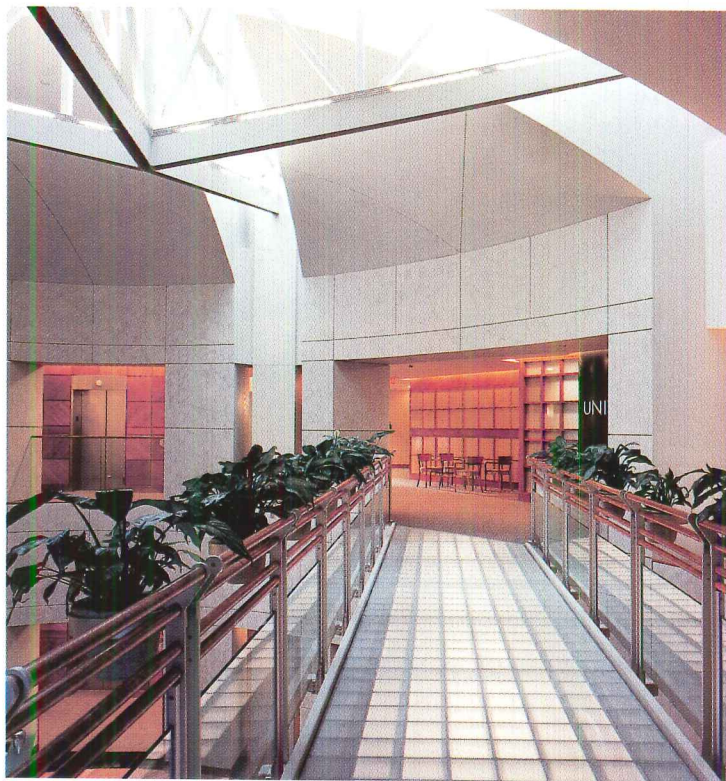
Skylights trace the top chords of the trusses, which support the ceiling and roof of the lobby, allowing daylight to enter the space. The glass-block floor of the bridge is illuminated by simple fluorescent strips fitted with 3500K high-color-rendering lamps. These are mounted in a perforated, bent-steel enclosure that hides the strips as well as acts as a reflector (left, right, and below).
