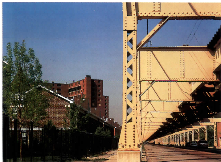
New low-rise and old high-rise buildings at Henry Horner sit along the El line.
