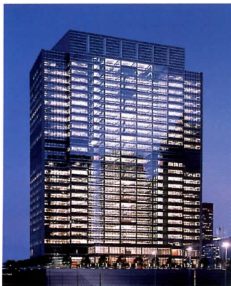
The Blue Cross Blue Shield of Illinois headquarters (above) has atria located on every fourth floor. These are illuminated by fluorescent uplights. MR-16s built into the canopy structure light the building’s entry.
